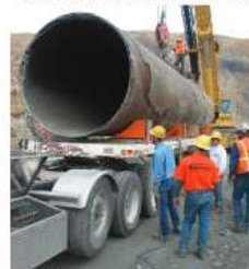
A portion of AA-1 pipeline had to be removed after the 2000 landslide.
